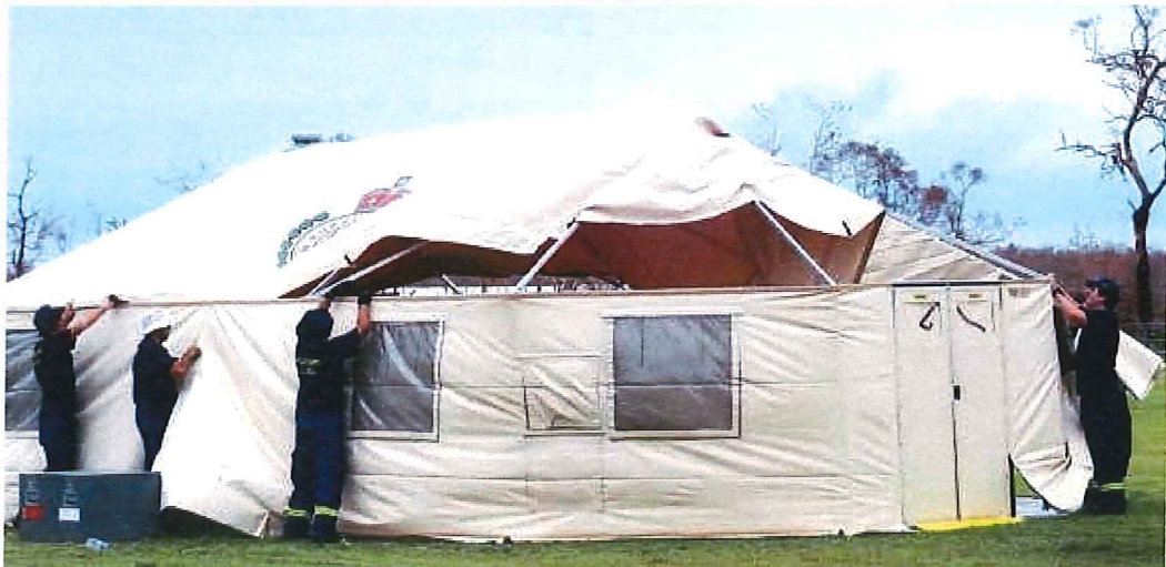
Galiwin'ku, Camp Elcho – shelter construction.
