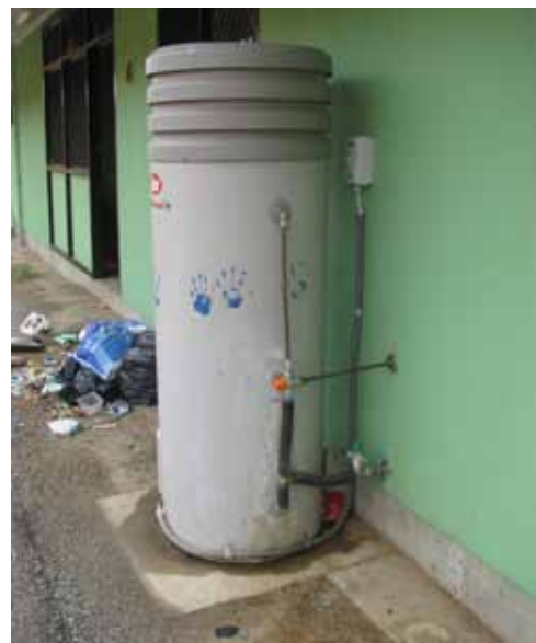
Figure 17 Heat pump hot water system
