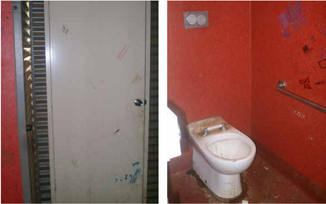
Figure 19 Prefabricated modular ablution & laundry block
