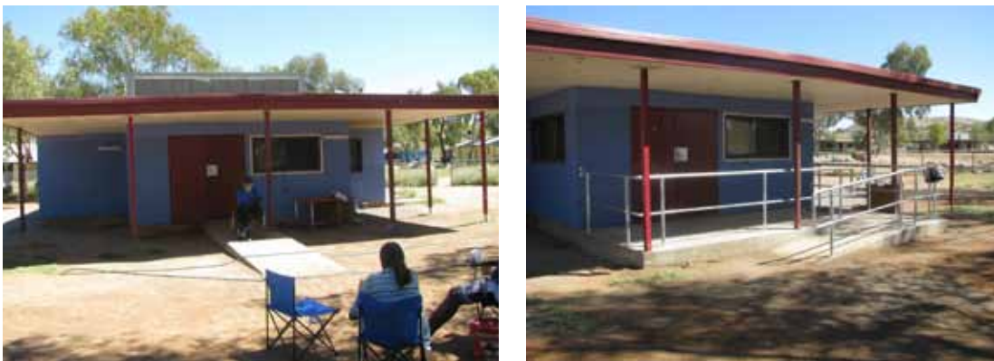
Figure 23 Modifications for accessibility; before (left) after (right)
