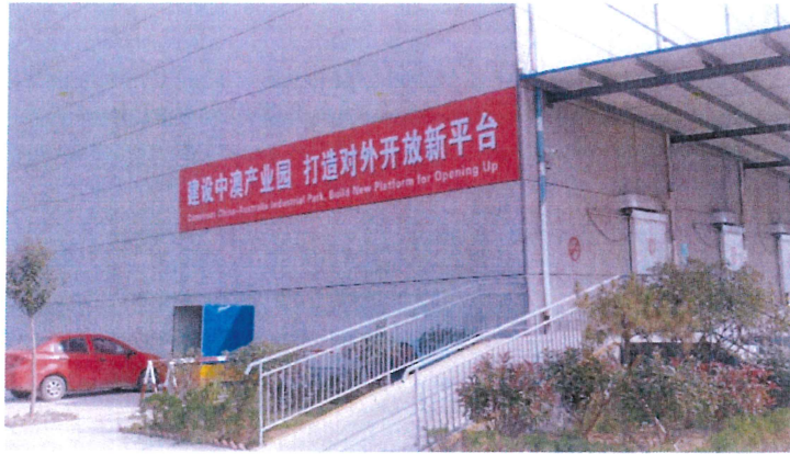
New refrigerated bonded storage facilities in Rizhao
