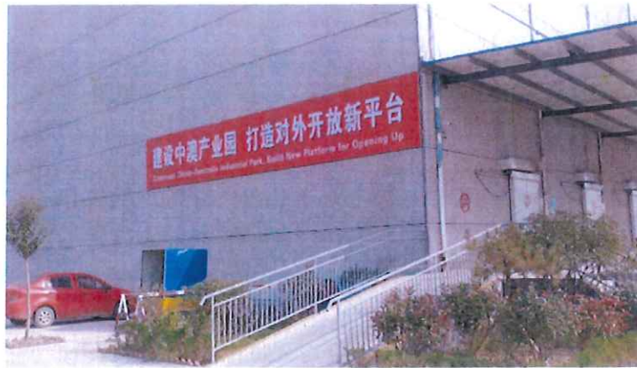
New refrigerated bonded storage facilities in Rizhao
