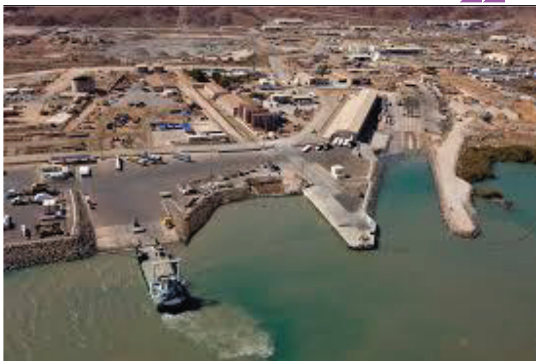
FIGURE 2.4 TOLL DAMPIER MARINE SUPPLY BASE SLIPWAY
