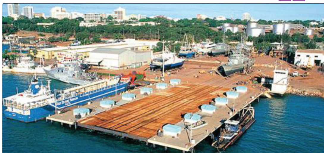
FIGURE 2.1 PEARL MARINE ENGINEERING – SYNCHROLIFT AND SHIPYARD
