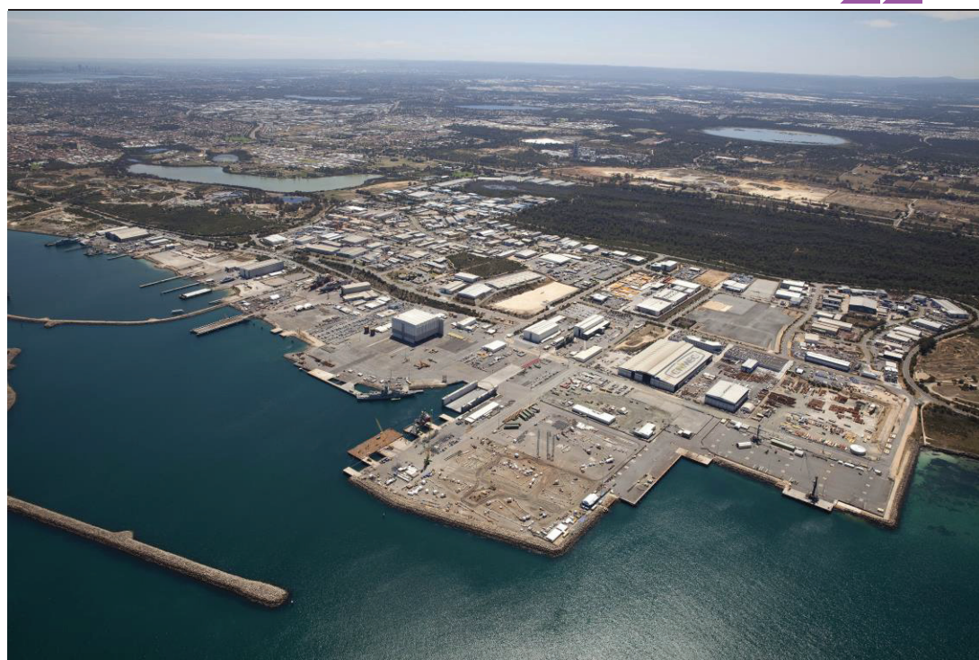
FIGURE 2.2 AMC COMMON-USER FACILITY, HENDERSON, W.A.
