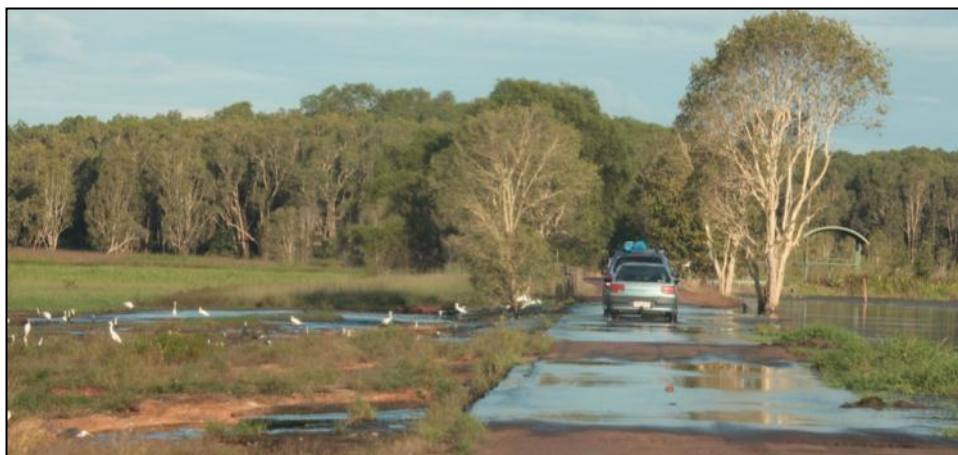
The elevated dam wall at Fogg Dam provides a raised, single-lane sealed road along which visitors can drive (Photo: © Michael J Barritt)
