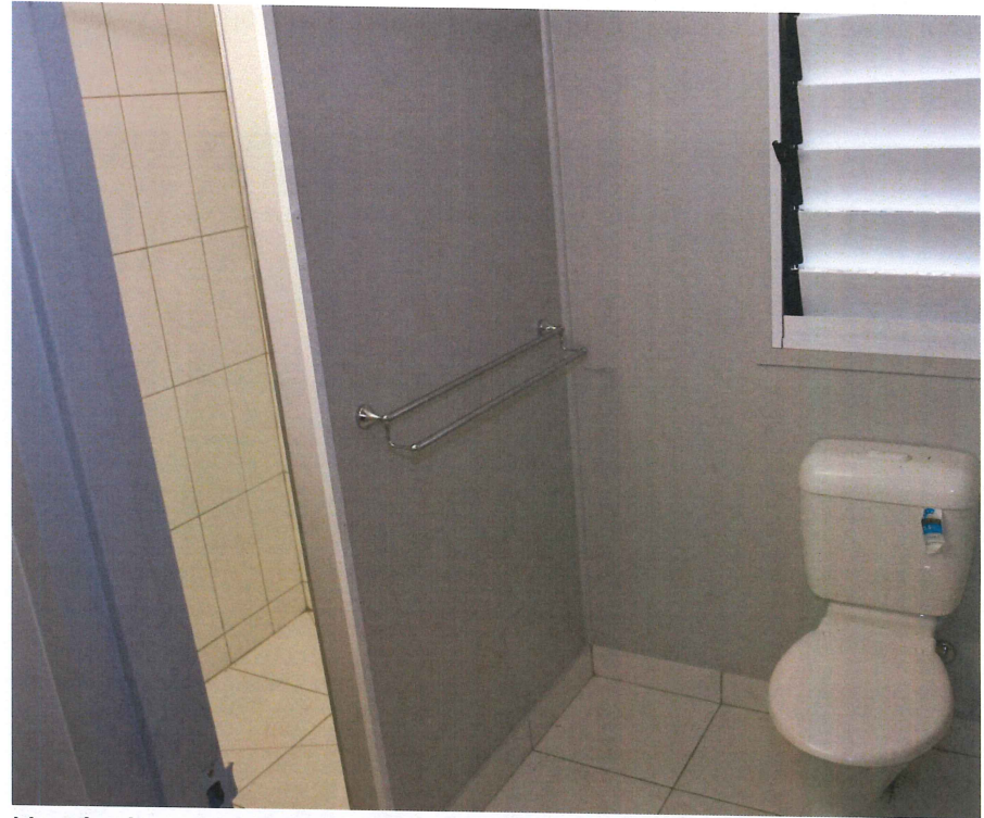
New bathroom at House 4
