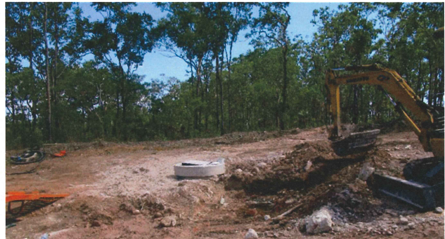
Works taking place in Johnston connecting the tunnel and pipe from PIV to the main sewerage network
