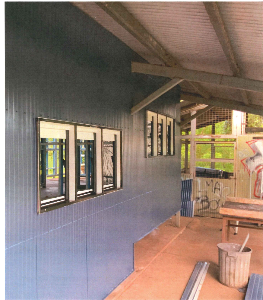
Progress work at House 9
