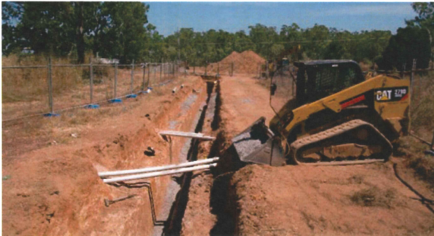
Infrastructure works taking place in PIV
