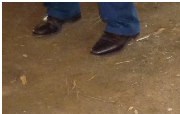
Damaged floor in house to be refurbished, Nguiu, 2 February 2010
