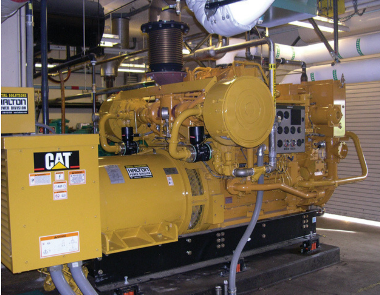
Gresham would like to increase its CHP capacity with another unit Source: City of Gresham
