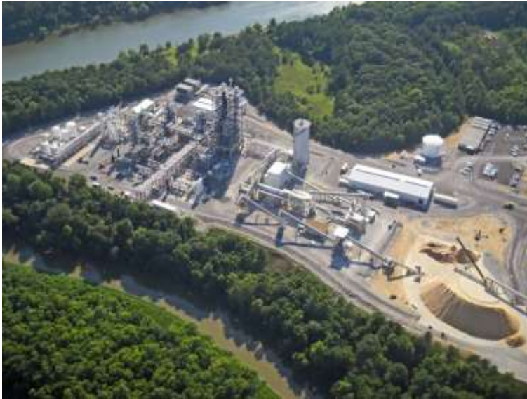
Figure 12: KiOR plant in Mississippi (source: KiOR)
