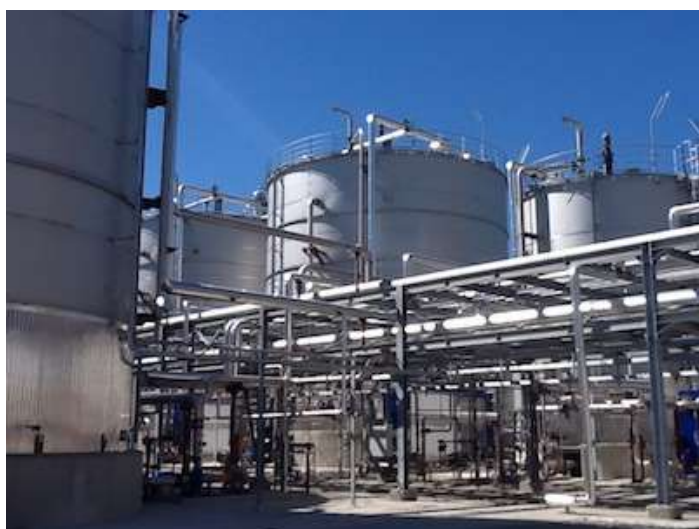
Figure 14: Beta Renewables Ethanol Plant in Crescentino, Italy
