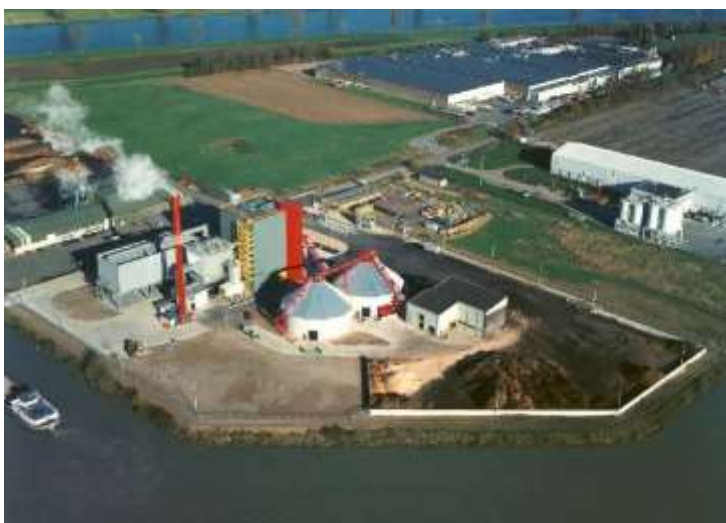
Figure 8: Aerial Photo of Cuijk 25 MW power plant (source Essent Energy)
