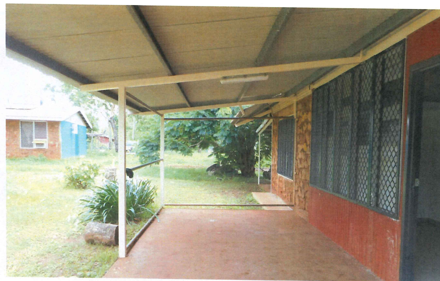
After photo - front verandah
