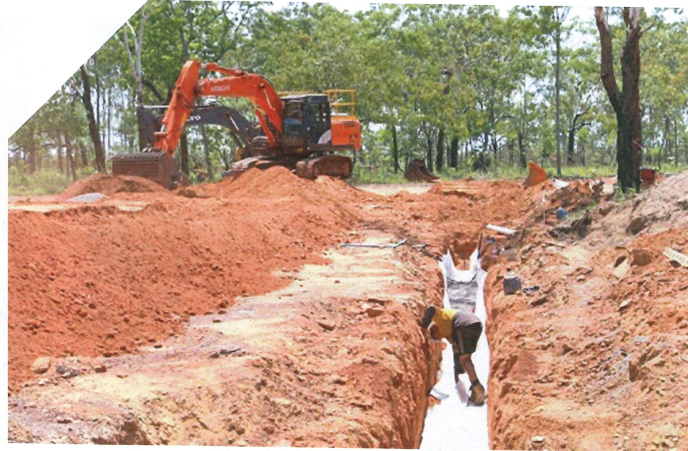
Subdivision work underway at Wadeye
