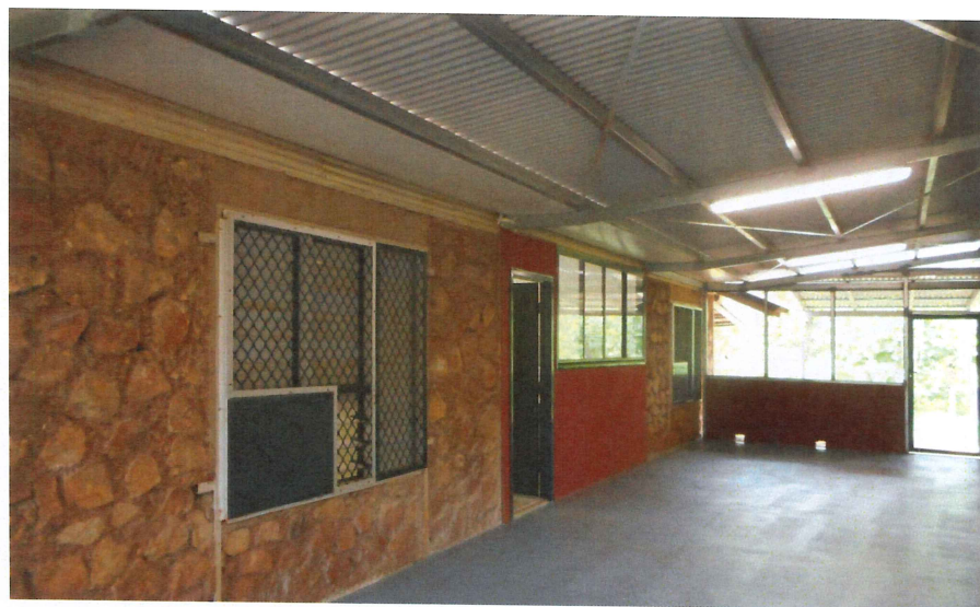
After photo - house to store room
