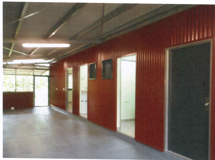
After photo - house to store room
