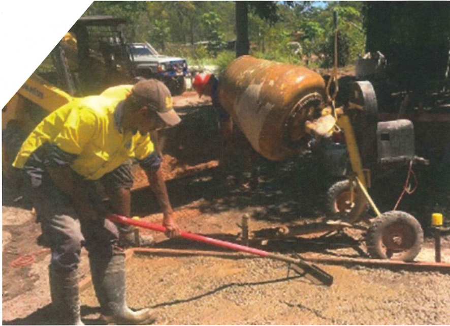
A worker laying a slab for Room to Breathe work at Milikapiti
