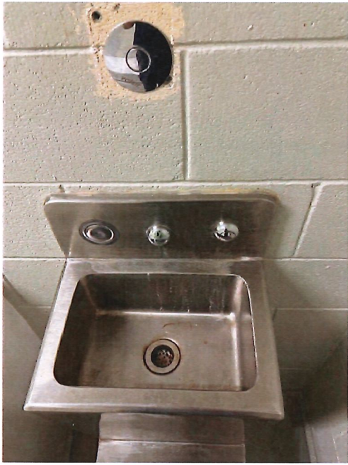
Figure 9 – Water bubbler and basin in the Alice Springs Watch House.
