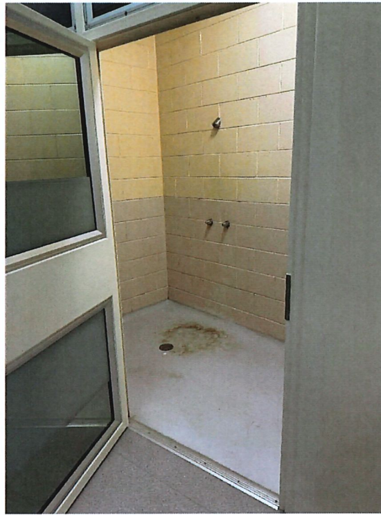
Figure 16 - Shower internal at the Palmerston Watch House.
