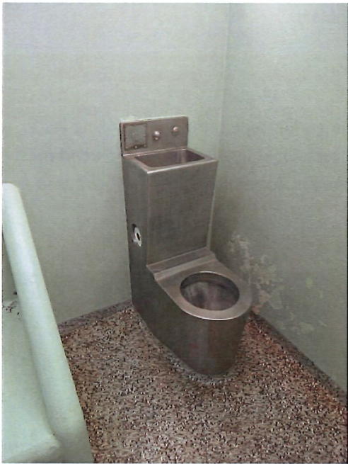
Figure 11 – Combined toilet and water basin in the Katherine Watch House.
