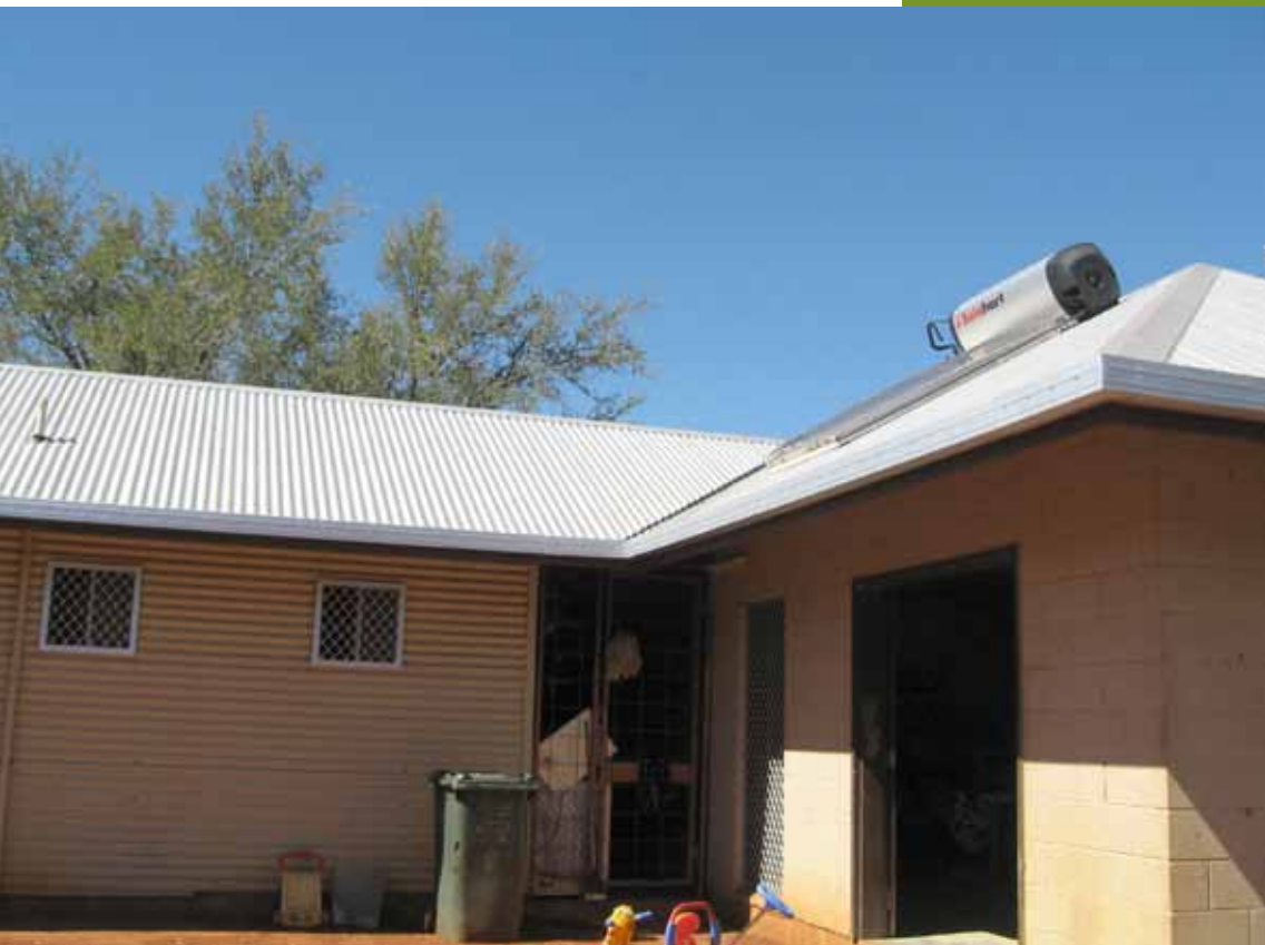
Housing refurbishments at Elliott
