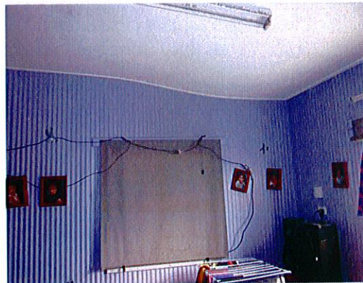
Item 2: Sagging ceiling lining in living room may indicate roof damage.
