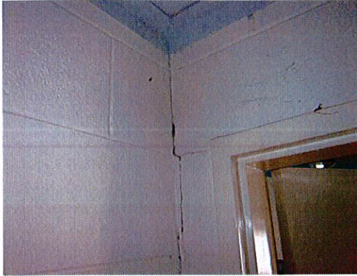
Item 5: Crack in wall adjacent to WC door.
