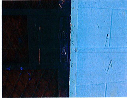
Item 6: Broken screen door handle makes safe entry an egress difficult.
