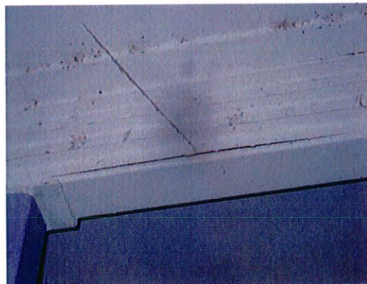
Item 9: Gaps between ceiling and beam.
